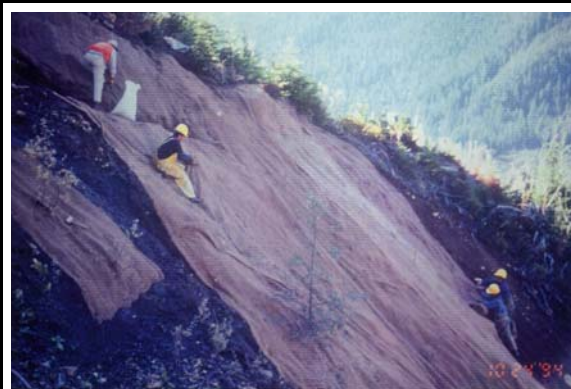
Slope Stability Matting to Reduce Erosion
