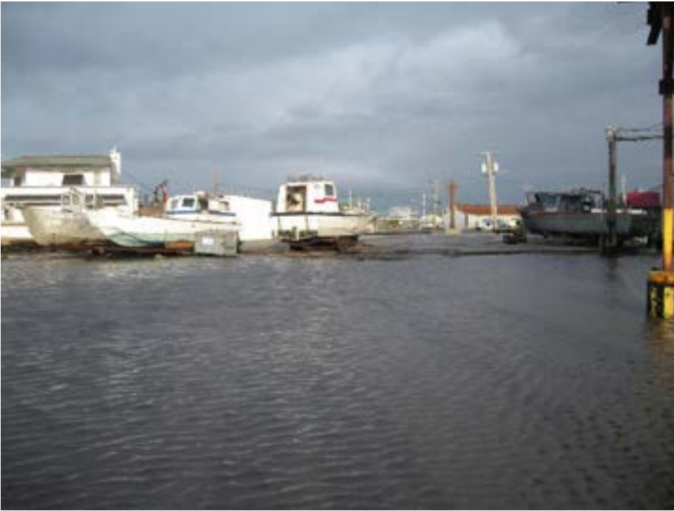
Coastal flooding at Gooseberry Point.
