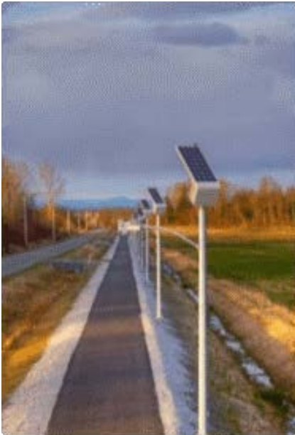
The Haxton Way Pedestrian Pathway is a 2-mile trail connecting the Silver Reef Casino to Kwina Road. It runs parallel to, but completely separate from, Haxton Way to create a safe route for pedestrians and cyclists. In 2011, solar-powered lighting was installed along the pathway as an added safety feature.
