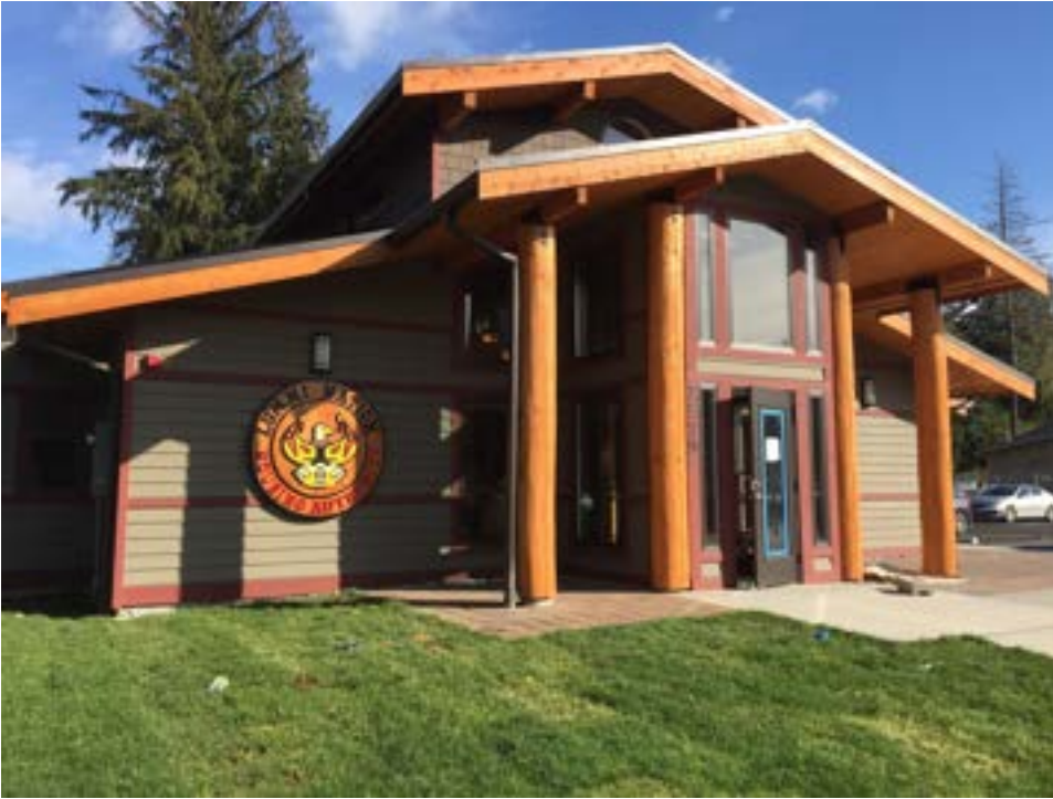
Lummi Nation Housing Authority administration building.
