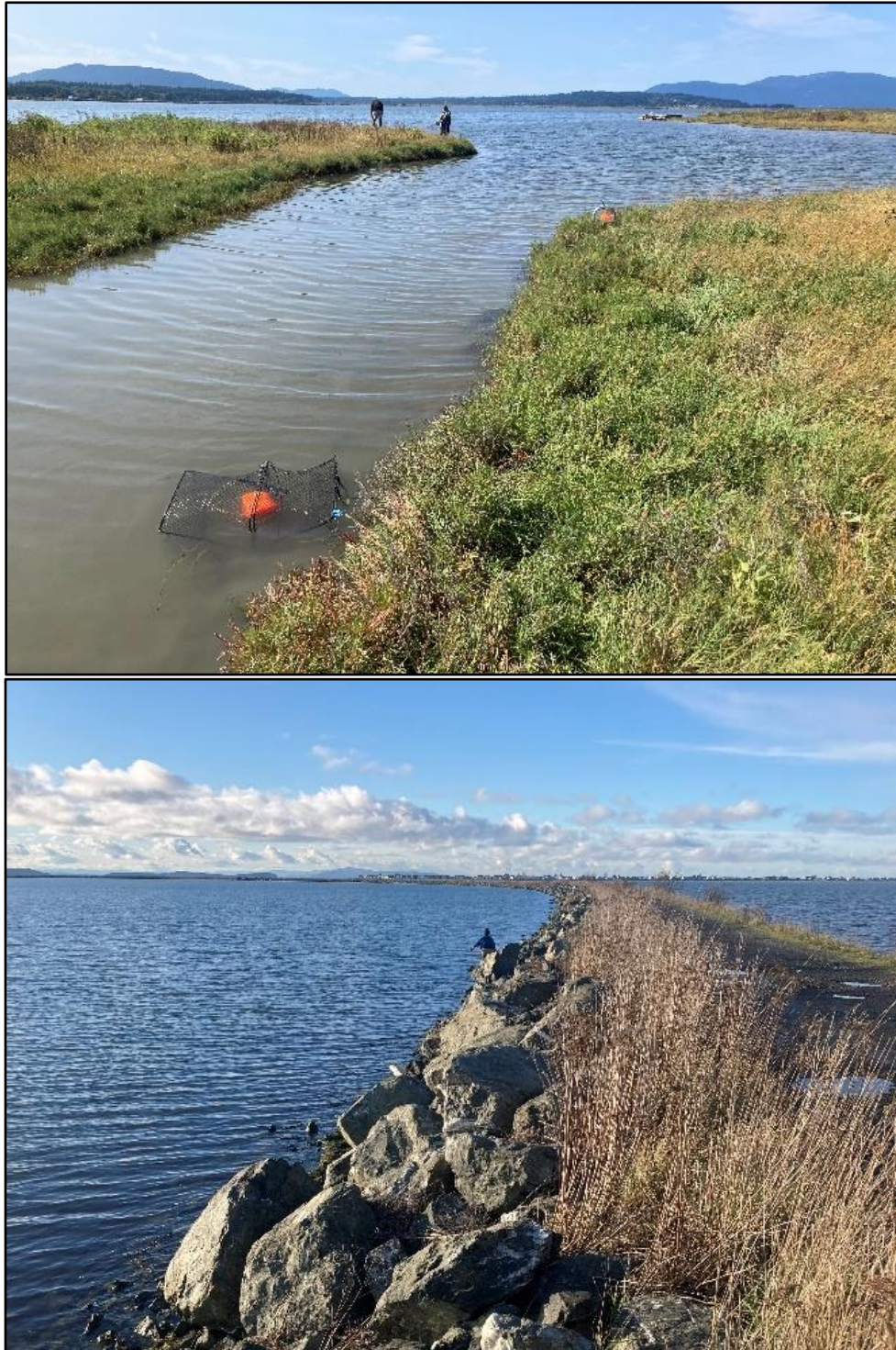
Figure 2. Shoreline types along the north central shoreline of Lummi Sea Pond (top) and the boulder dike wall (bottom); pictured on top are Elias Plaster and Delaney Adams (LNR), photo credit Bobbie Buzzell.
