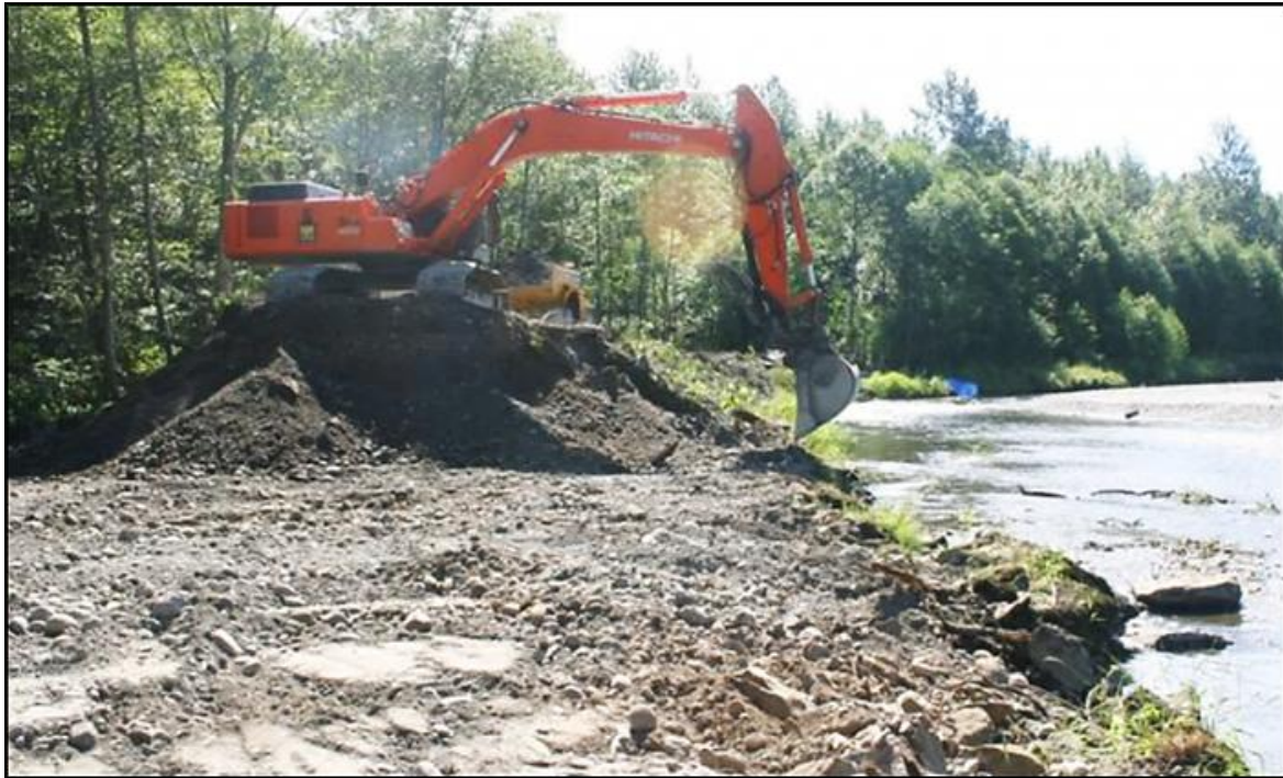
Figure 92: Levee removal as a part of the Lower Hutchinson Project.
