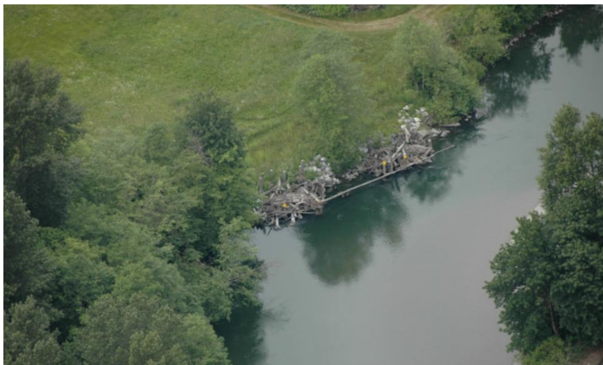
Figure 116: Hardscrabble logjams build into an existing riprapped bank.
