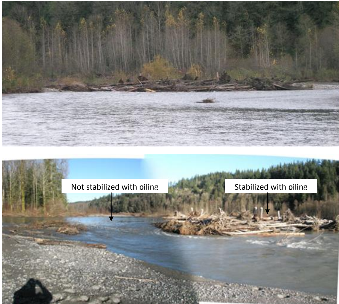
Figure 80: A natural logjam that was partially stabilized with piles. The stabilized portion persisted through the high flow, while the rest of the logjam was transported downstream.
