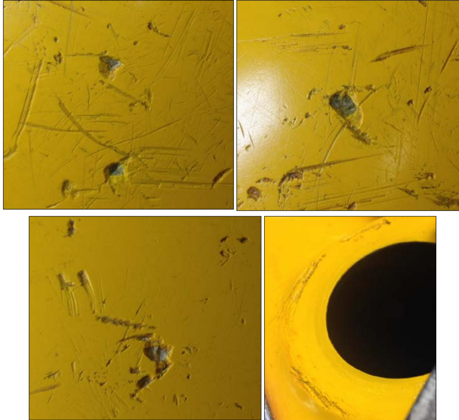
Numerous gouges, some into the fiberglass
