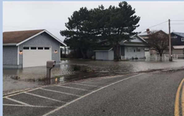
Coastal Flooding at Gooseberry Point in 2022
