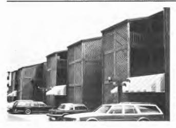
Figure 3.32. The diagonal battens used to enclose the stairwells for protection provide an aesthetically appealing screen-textural affect. The colored awnings also add a necessary highlight to an otherwise colorless exterior. Notice also the pole light fixture.
