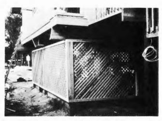
Figure 4.54. Breakaway Walls
