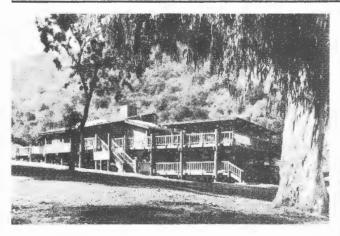
Figure 3.25. This wood structure successfully uses the same material throughout the building—foundation, structure, treatment of railings, wall, and roof material, as well as connection and anchorage details. The design honestly expresses the structure, foundations and other building elements. While it is obvious this is an elevated structure, it still feels very much a part of the site. The foundation members are also integrated well with the building itself (see also Figures 3.54 to 3.57).
