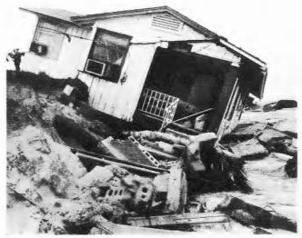
Figure 2.3. Erosion Caused This Foundation to Collapse.
