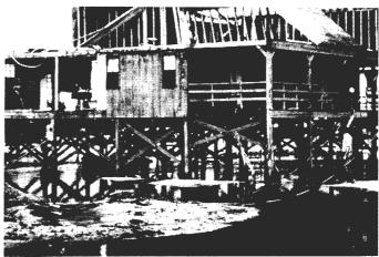
Figure 4.23. Diagonal Bracing
