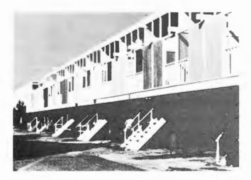
Figure 3.30. The exterior treatment of this development adds visual appeal to a development that could otherwise be quite monotonous. The exterior colored panels with white structure and coordinated interior panels provide interest, as does the simple treatment of balconies with a variety of planes, panels, railing and roof trellis members.
