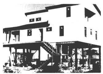
Figure 4.14. Pile Foundations
