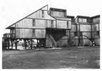
Figure 4.4. Elevation by Posts
