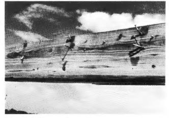
Figure 4.26. Toe Nailing Provides Limited Pull-Out Resistance
