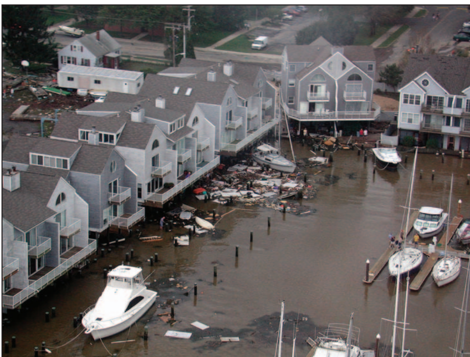
Figure 4-21. Condominiums built along the shoreline at the mouth of the Susquehanna River on the Chesapeake Bay were subjected to flood-borne debris after Hurricane Isabel (Havre de Grace, MD, 2003)
