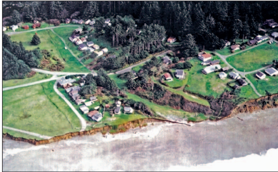
Figure 4-19. As buildings in this Humboldt County, CA, community are threatened by bluff erosion along the Pacific Ocean, they are moved to other sites on the jointly owned parcel
