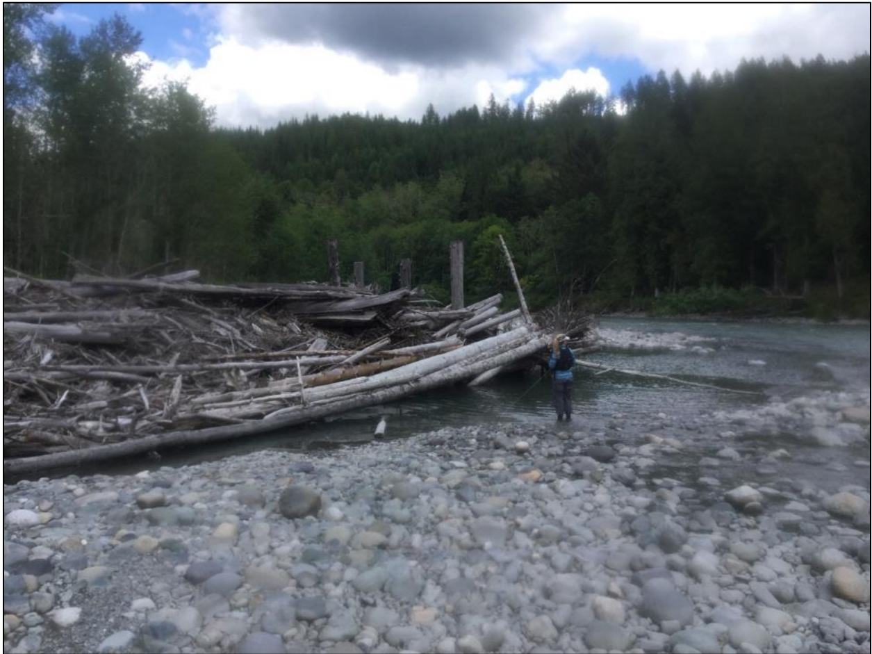
Figure 50. ELJ disconnected from the mainstem channel within the Cavanaugh Island project area. While a scour pool is forming when the jam is engaged with higher flows, the feature is disconnected from the main-channel flow during low flow conditions. The ELJ is located along the left bank near RM 16.8 and is the middle ELJ near the side-channel inlet location. The photo was taken on 6/28/18 with flow to the left.
