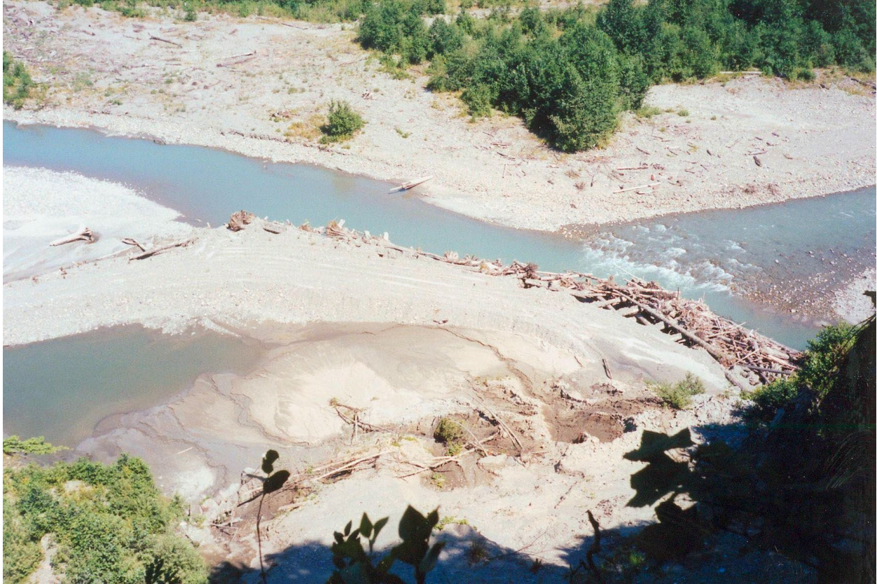
Figure 37. Sediment storage behind revetment in Larson's Phase 1 (Source: Maudlin 2005).
