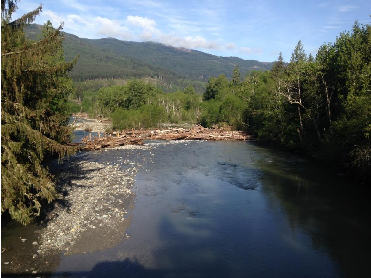
Figure 31. ELJ at Larson’s Phase 2 showing wood racking on jam.
