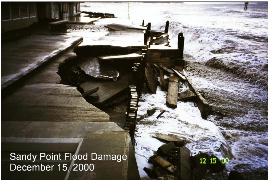
(b) Destroyed Bulkhead and Deck (Several Hours after Peak Waves)
