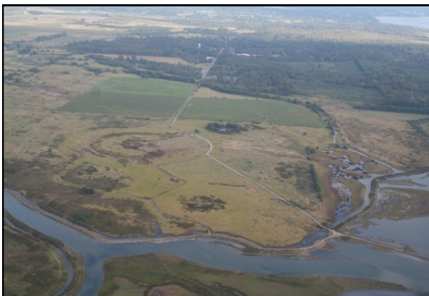
Blockhouse Site: Historic salt marsh areas in the Lummi River delta will be restored by re-establishing connection to marine waters and direct tidal influence.
